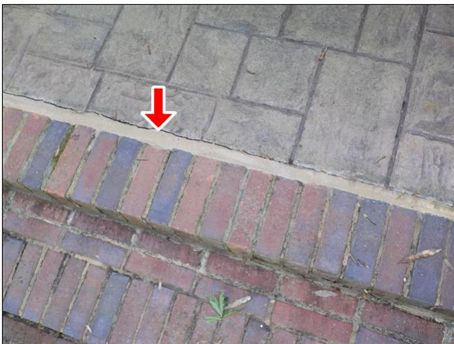
1.5 Item 8 Gap has been filled
